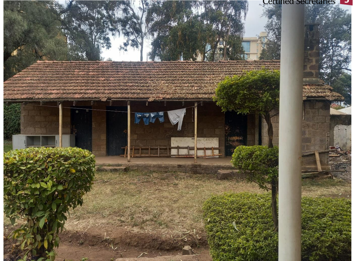
Photo 04: Proposed washrooms for the Semi-Permanent Training Facilities. (NB: To be renovated)
